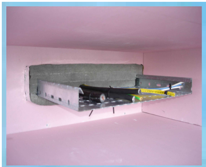
Cable Basket Fire Sleeve Installed in Partition
