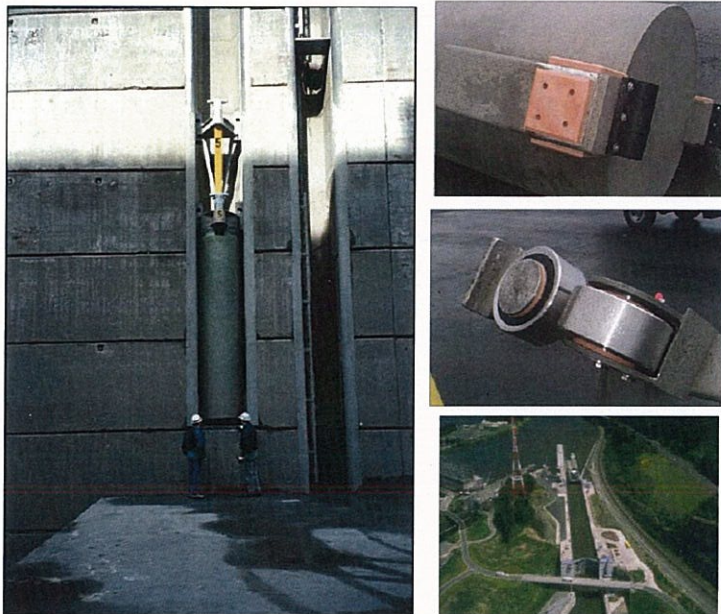
Bonneville Vertical Gate showing sliding pad and roller wheel bearing.
