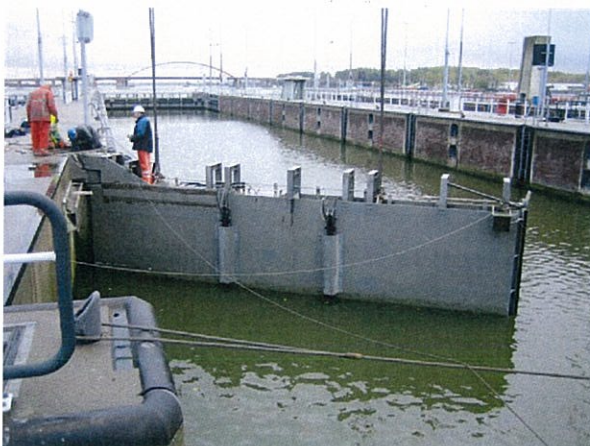
Gate showing upper hinge on left hand side.
